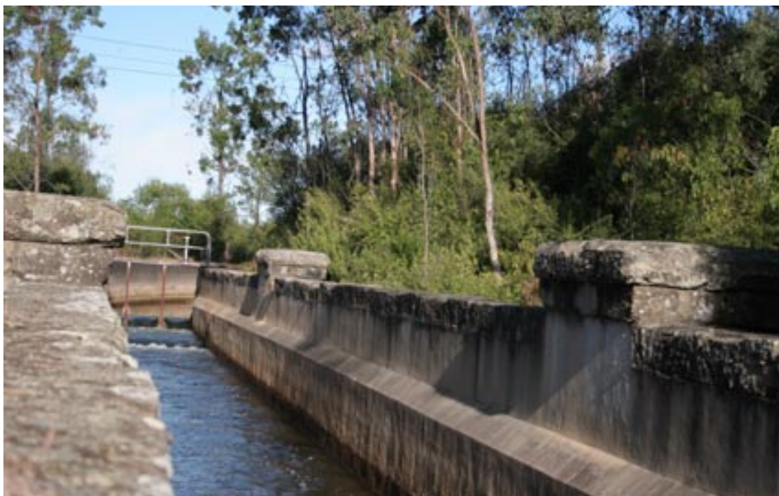
Unfiltered water is drawn from the on-site canal. Allen Powell
